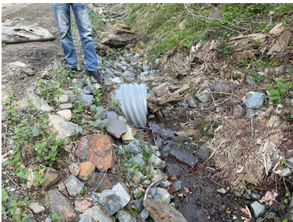
Lower culvert inlet
