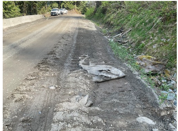
Geotextile on road
